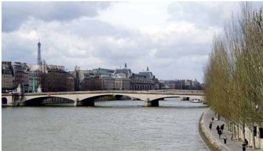
Figure 10 – UMDENSTOCK, Gustave, TOURRY, Georges, LANG, Henri, MORANE, Jacques, Paris, Pont du Carrousel, 1935-1939
